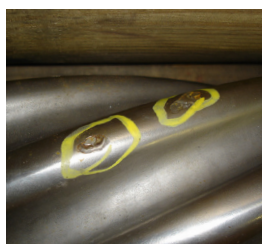
Damaged rotors are inspected prior to restoration.
